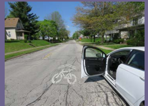
Image 6.3: Shared Lane Marking (Sharrow) placement outside of the "door zone" in Moline
