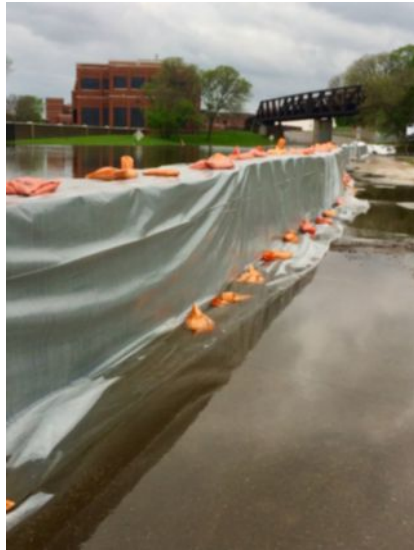
Figure 2.4 U.S. 67/River Drive, Davenport and Temporary Flood Barrier (2019)
