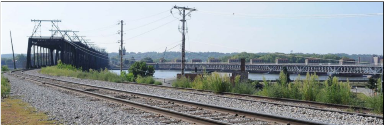
Existing Government Bridge and Dam 15 from Davenport Trainway | Source: HDR
