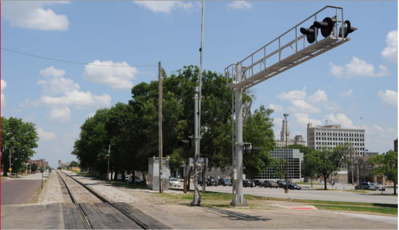
Western Avenue Crossing in Davenport | Source: HDR
