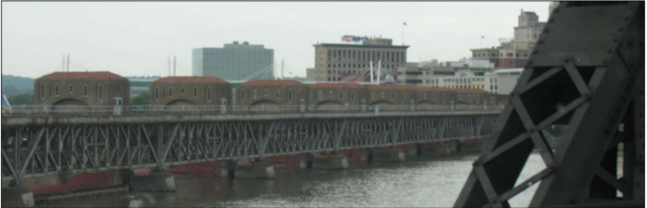
Existing Dam 15 from Government Bridge | Source: HDR
