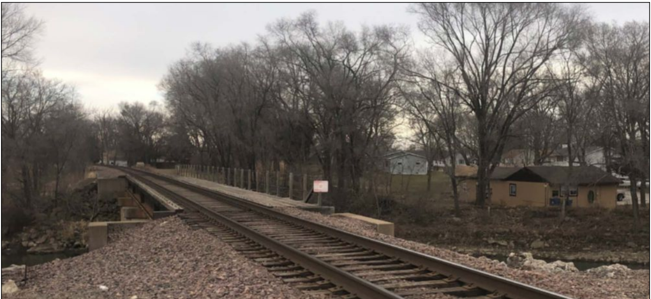
Existing CP Bridge over Duck Creek in Bettendorf, Iowa | Source: HDR
