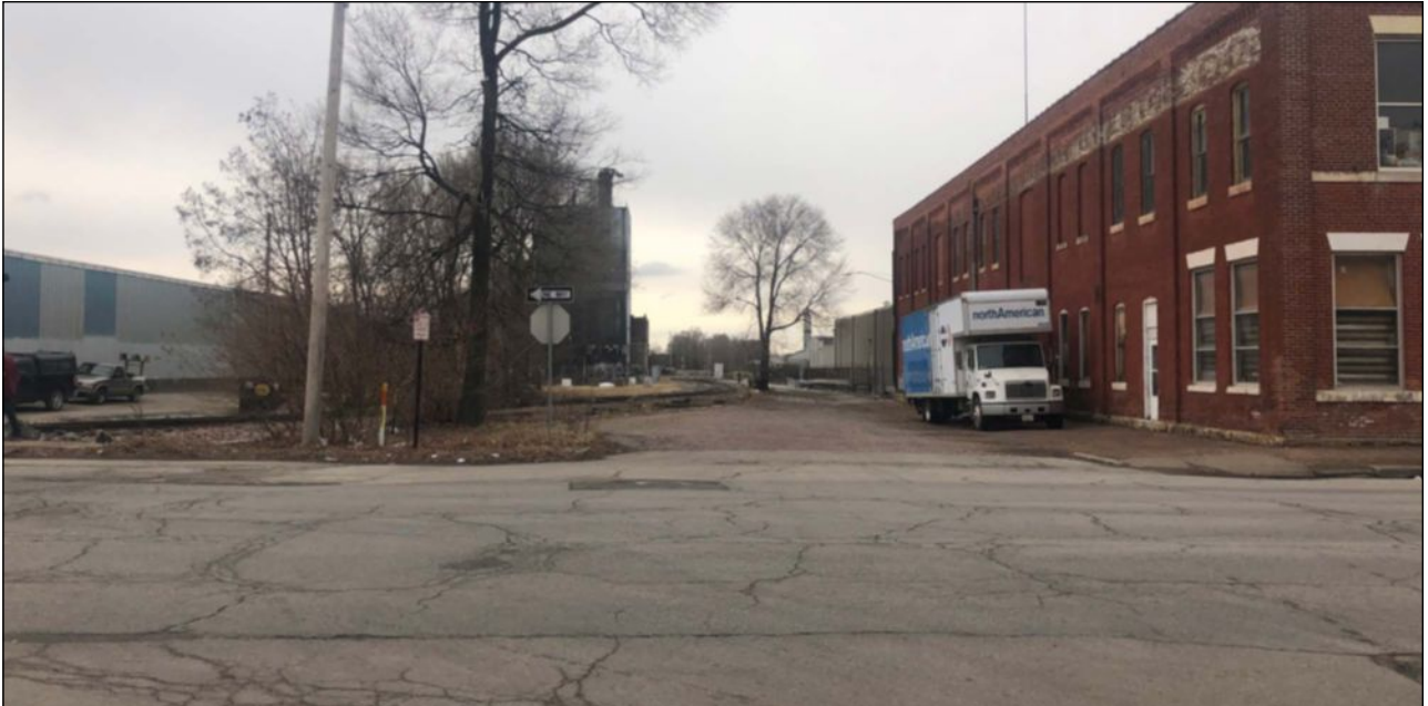
Existing Missouri Division Junction Interchange Track Looking South from 3rd Street | Source: HDR
