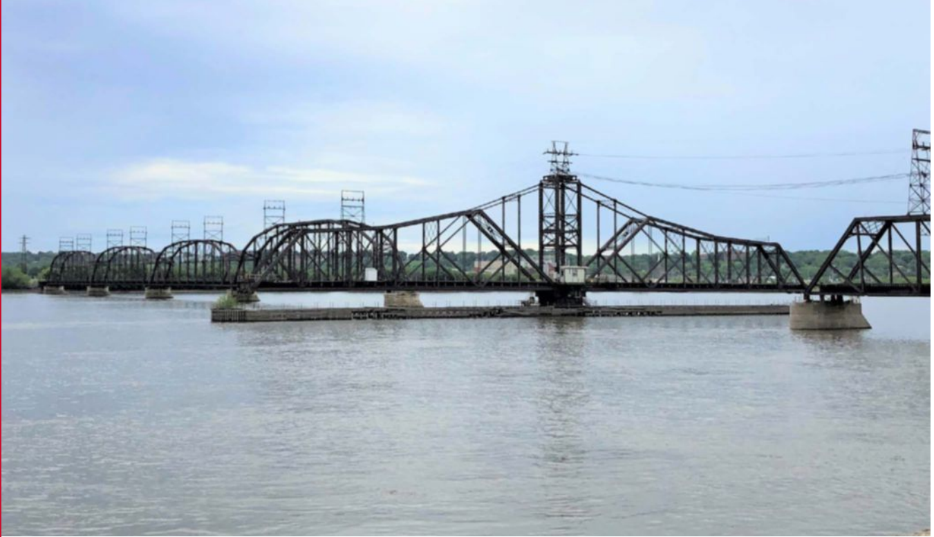
Existing Crescent Bridge | Source: HDR
