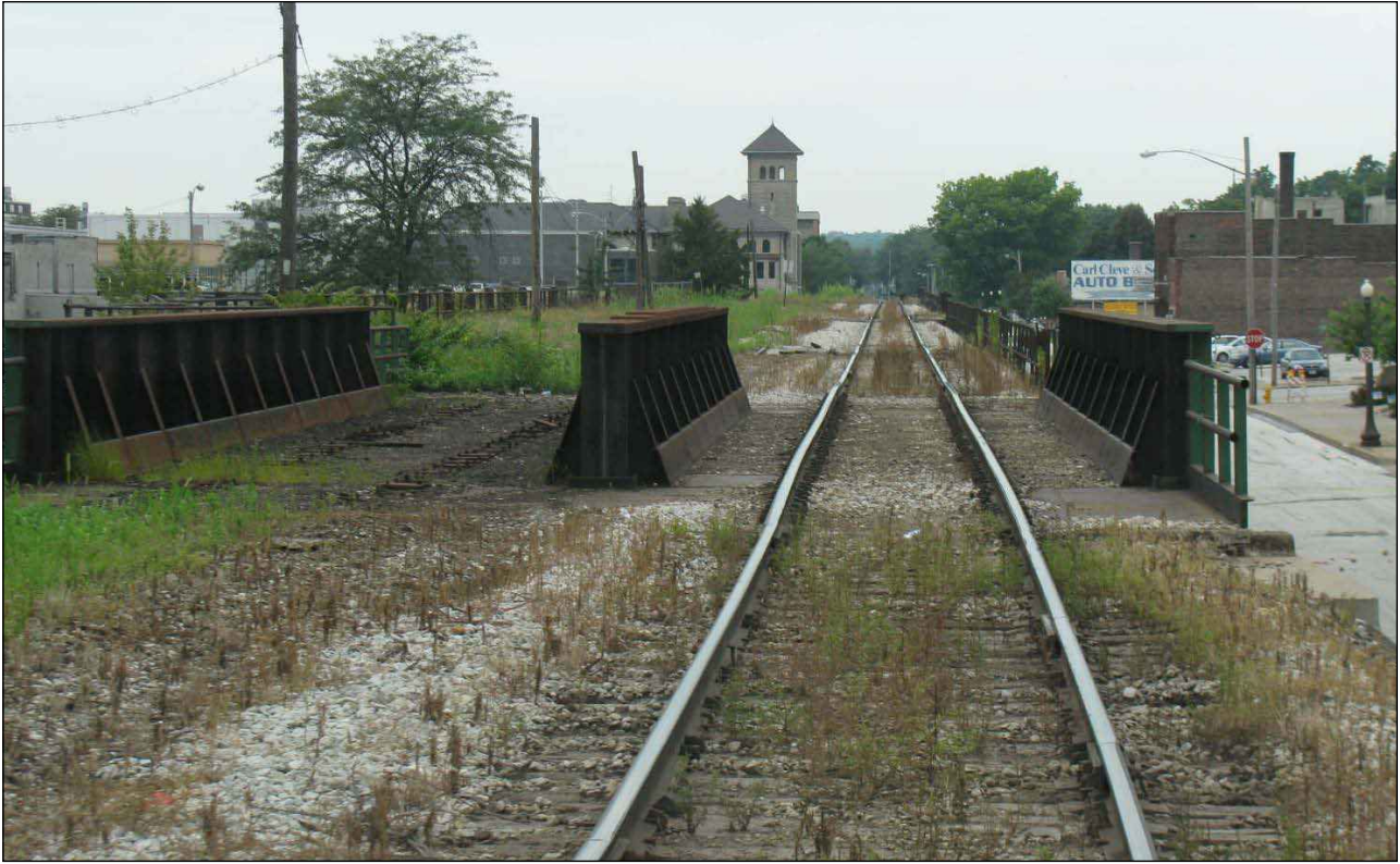
Existing Davenport Trainway Looking West from Brady Street | Source: HDR
