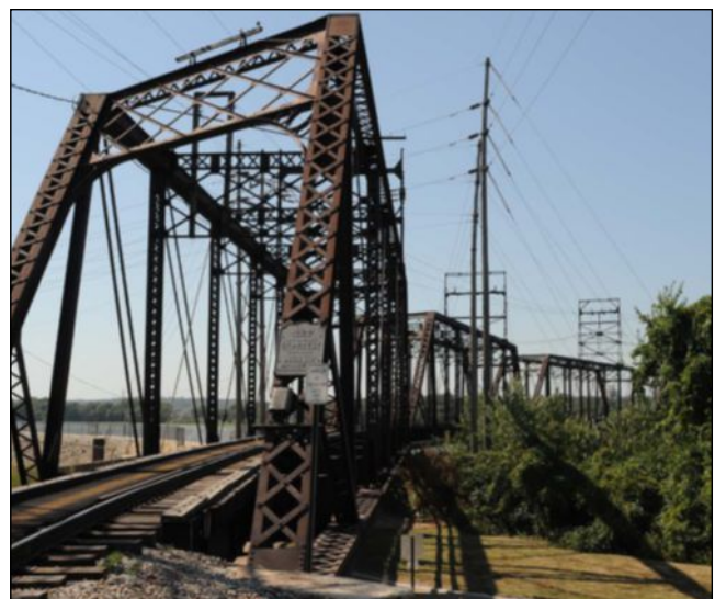
Existing Crescent Bridge | Source: HDR
