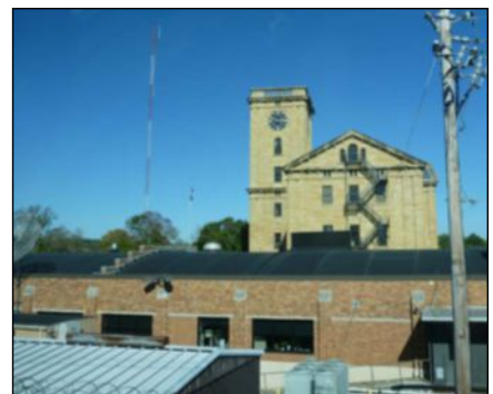
Historic Rock Island Arsenal Clock Tower | Source: HDR
