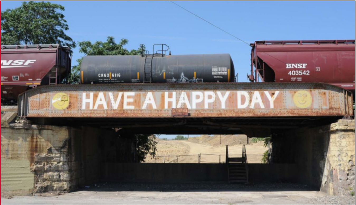
Former IAIS Bridge 180.6 in Rock Island | Source: HDR
