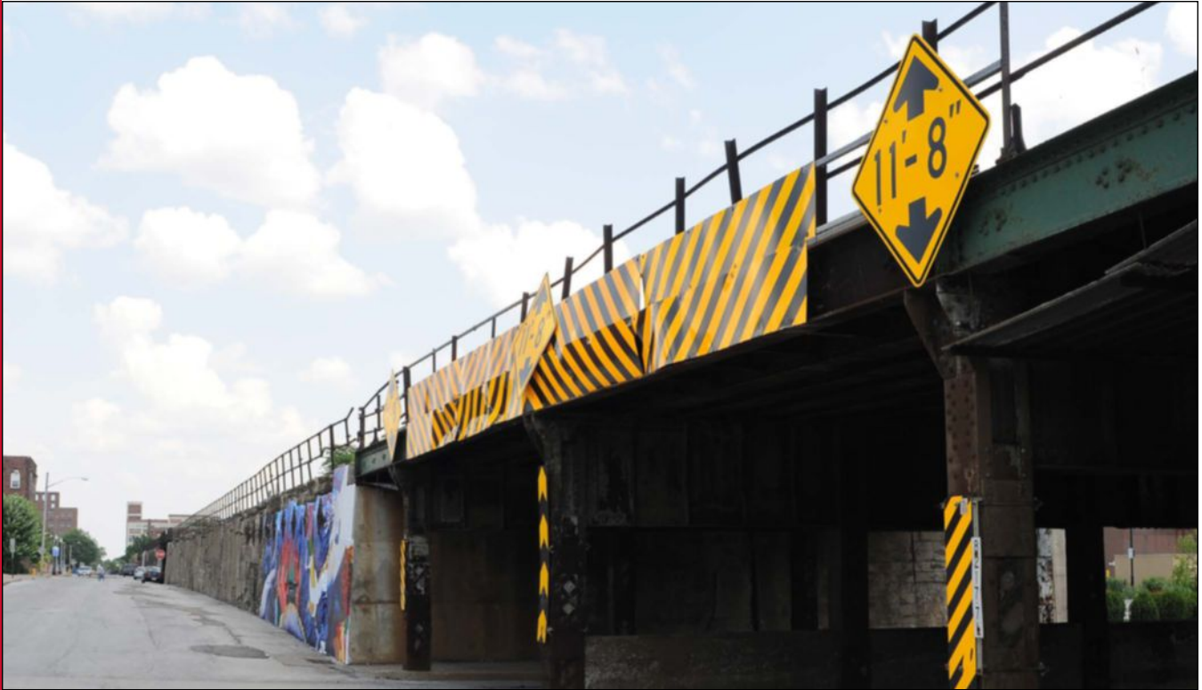
Harrison Street (U.S. Highway 61) Bridge on Davenport Trainway | Source: HDR
