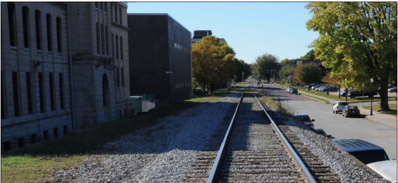
Existing Davenport Trainway between Ripley Street and Western Avenue | Source: HDR
