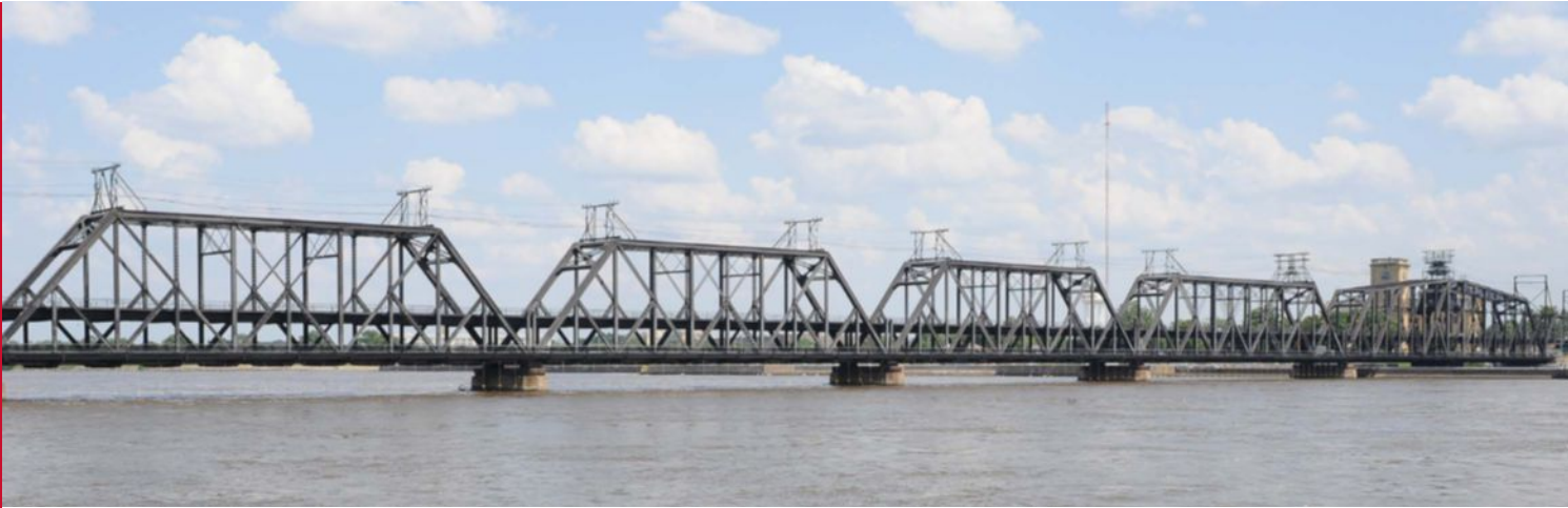
Existing Government Bridge | Source: HDR
