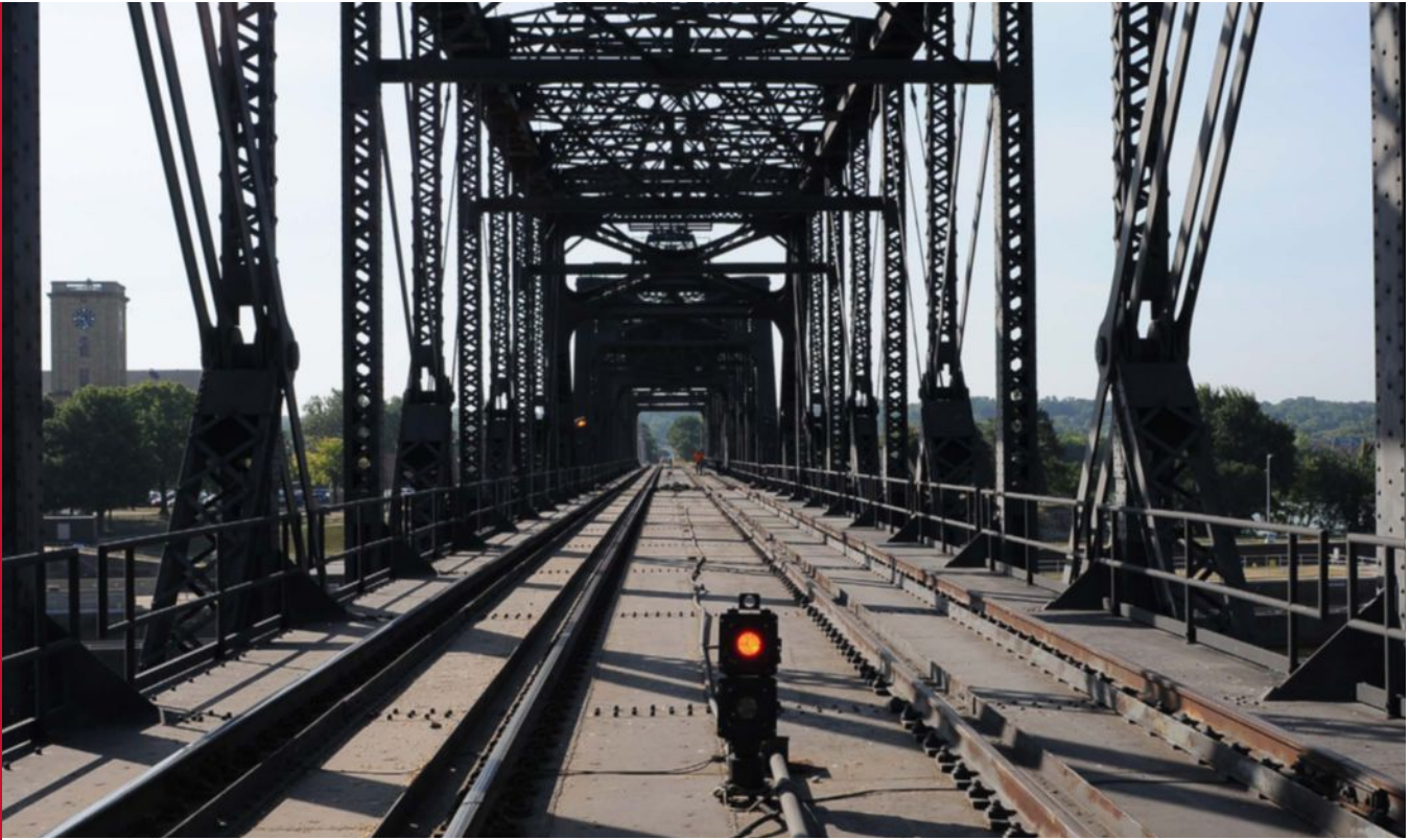
Existing Government Bridge | Source: HDR
