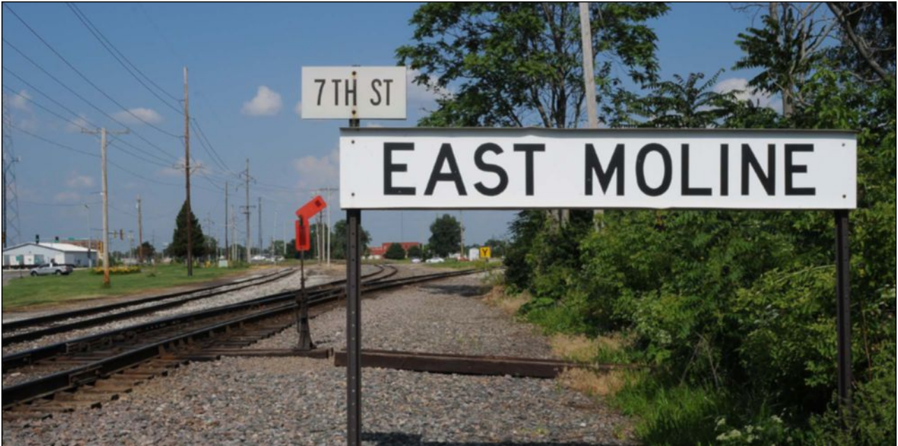
Existing 7th Street Interlocking in East Moline | Source: HDR
