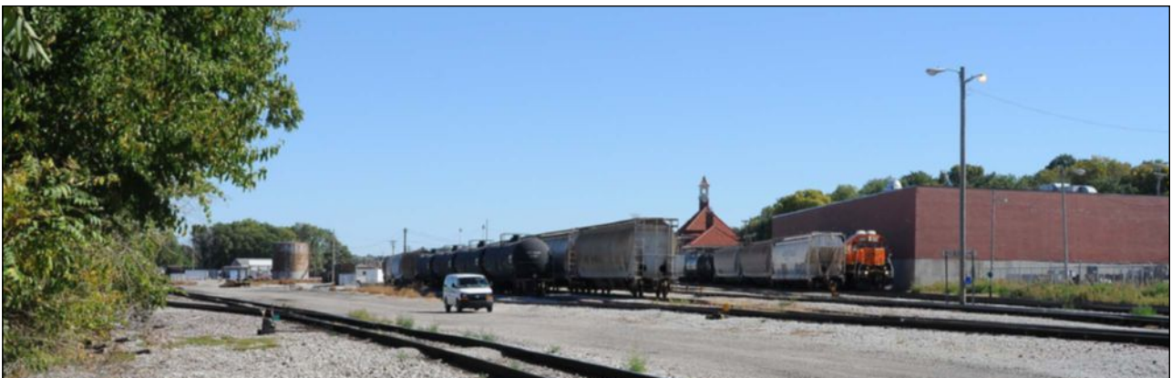
IAIS Rock Island Yard with BNSF Interchange | Source: HDR
