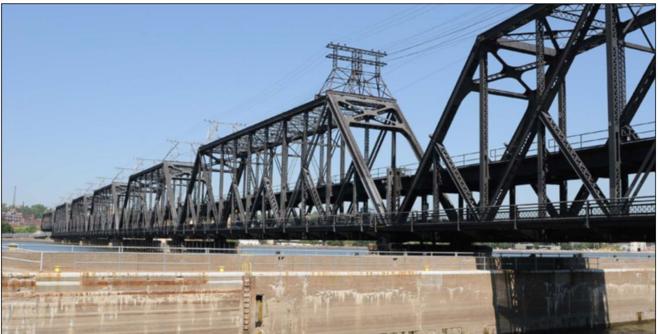
Existing Government Bridge at Lock 15 | Source: HDR
