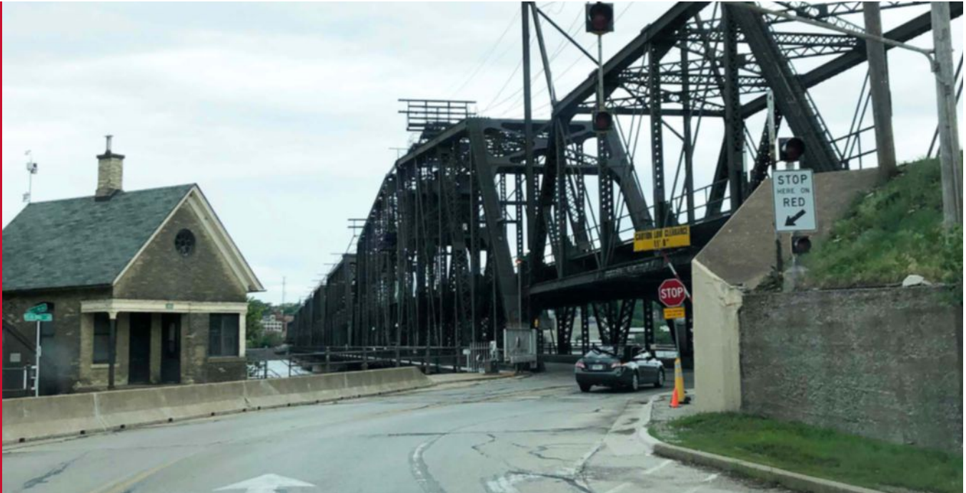
Arsenal Island Roadway Approach to Government Bridge River Crossing | Source: HDR
