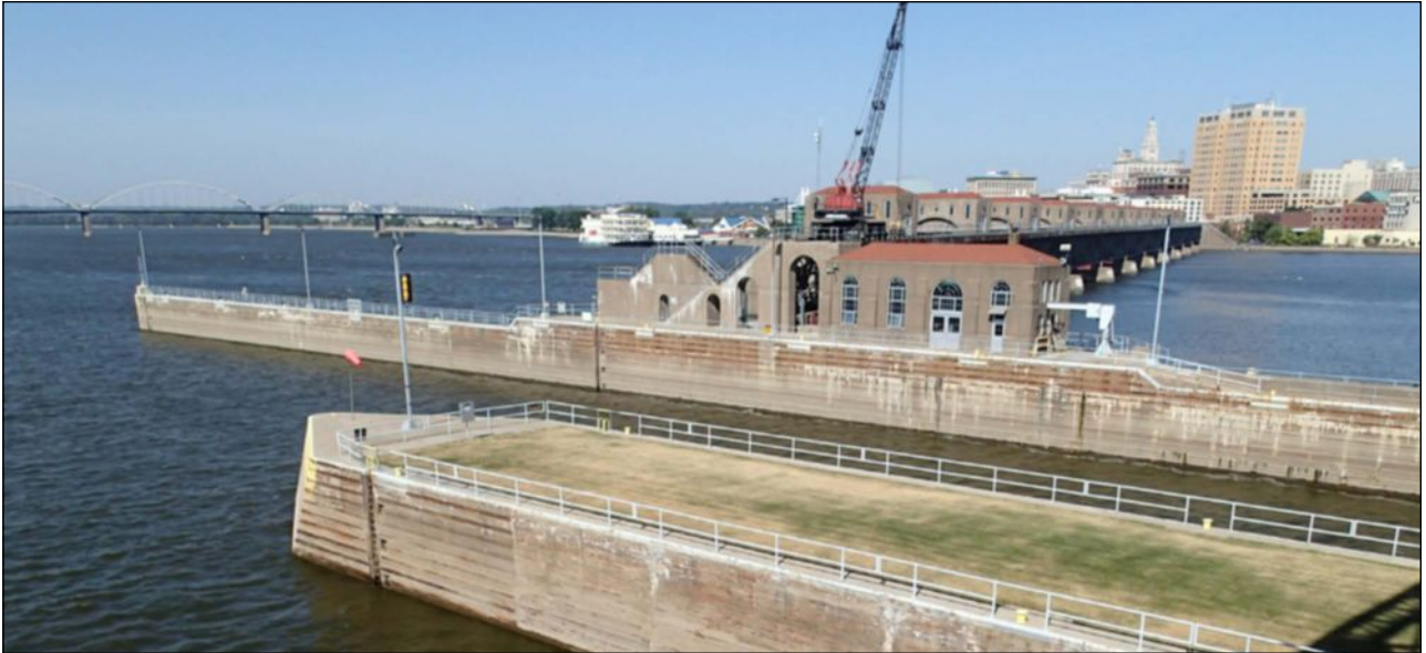
Harrison Street (U.S. Highway 61) Bridge on Davenport Trainway | Source: HDR
