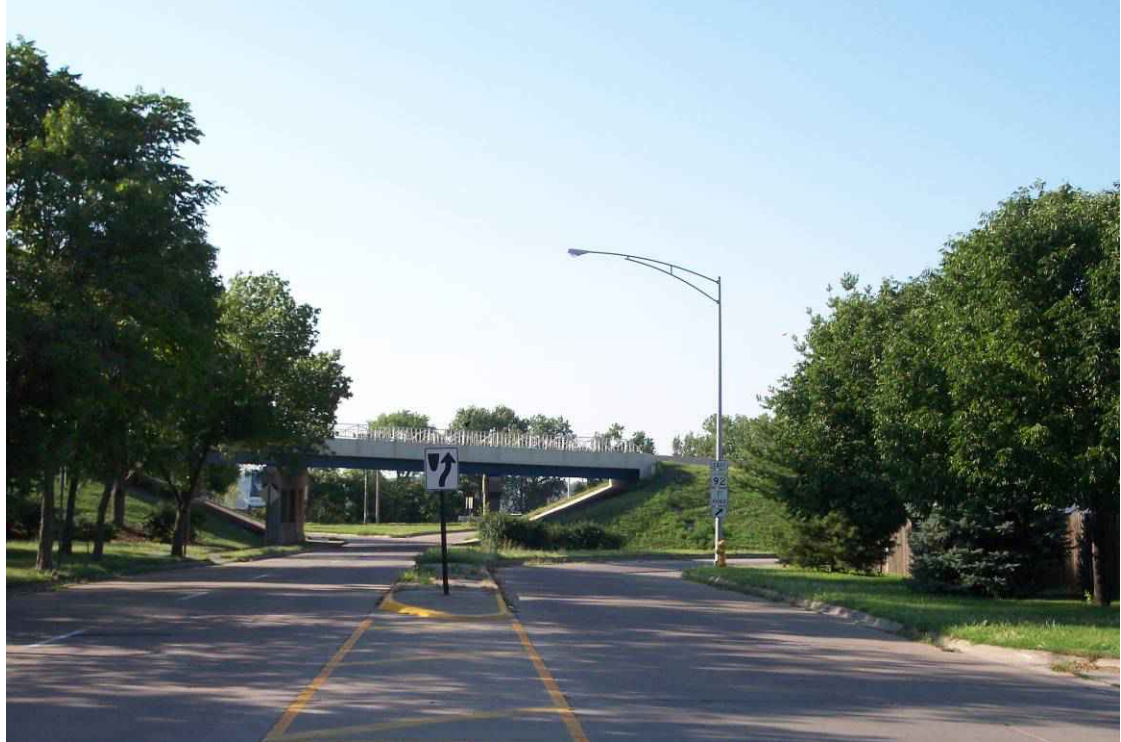
Existing 11 th Street Interchange – View looking north.
