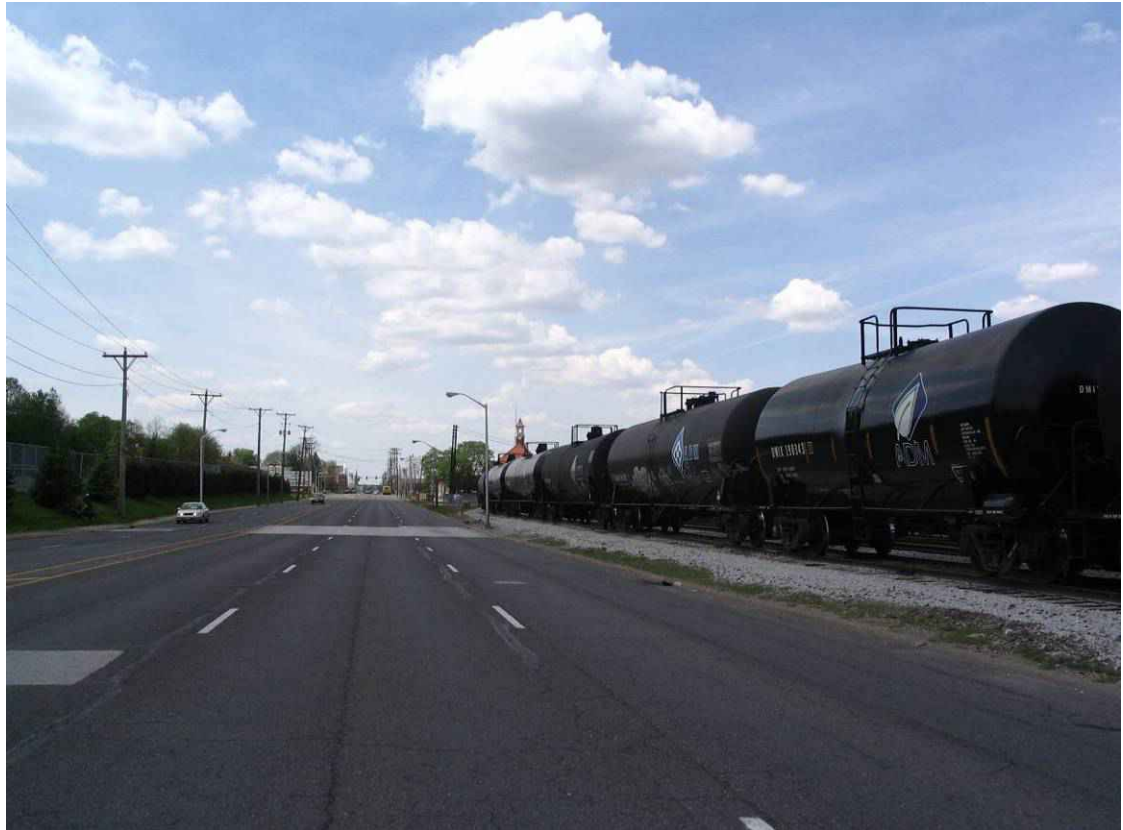
Existing 5 th Avenue – View looking west near 37 th Street.
