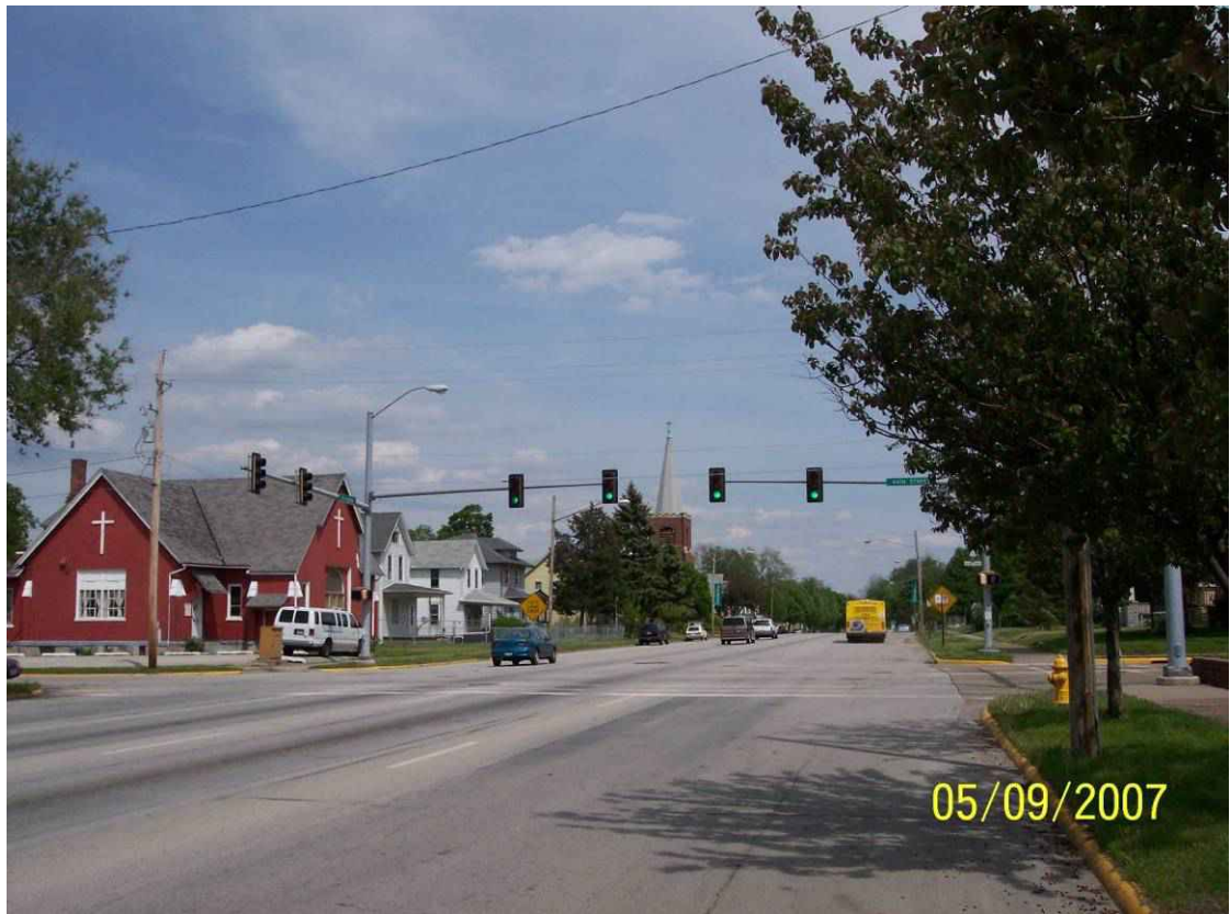
Existing 7 th Avenue – View looking east at 44 th Street.
