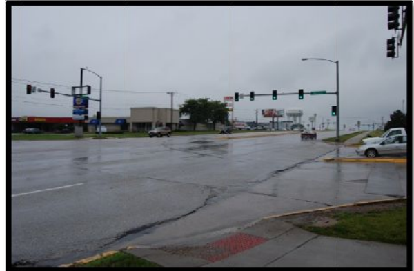
Figure 5.10 Photo- Main St. & Kimberly Rd. (Davenport)
