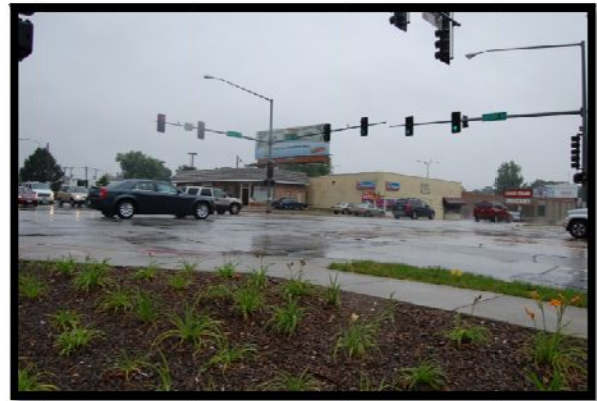
Figure 5.25 Photo- West Locust St. & Brady St. (Davenport)
