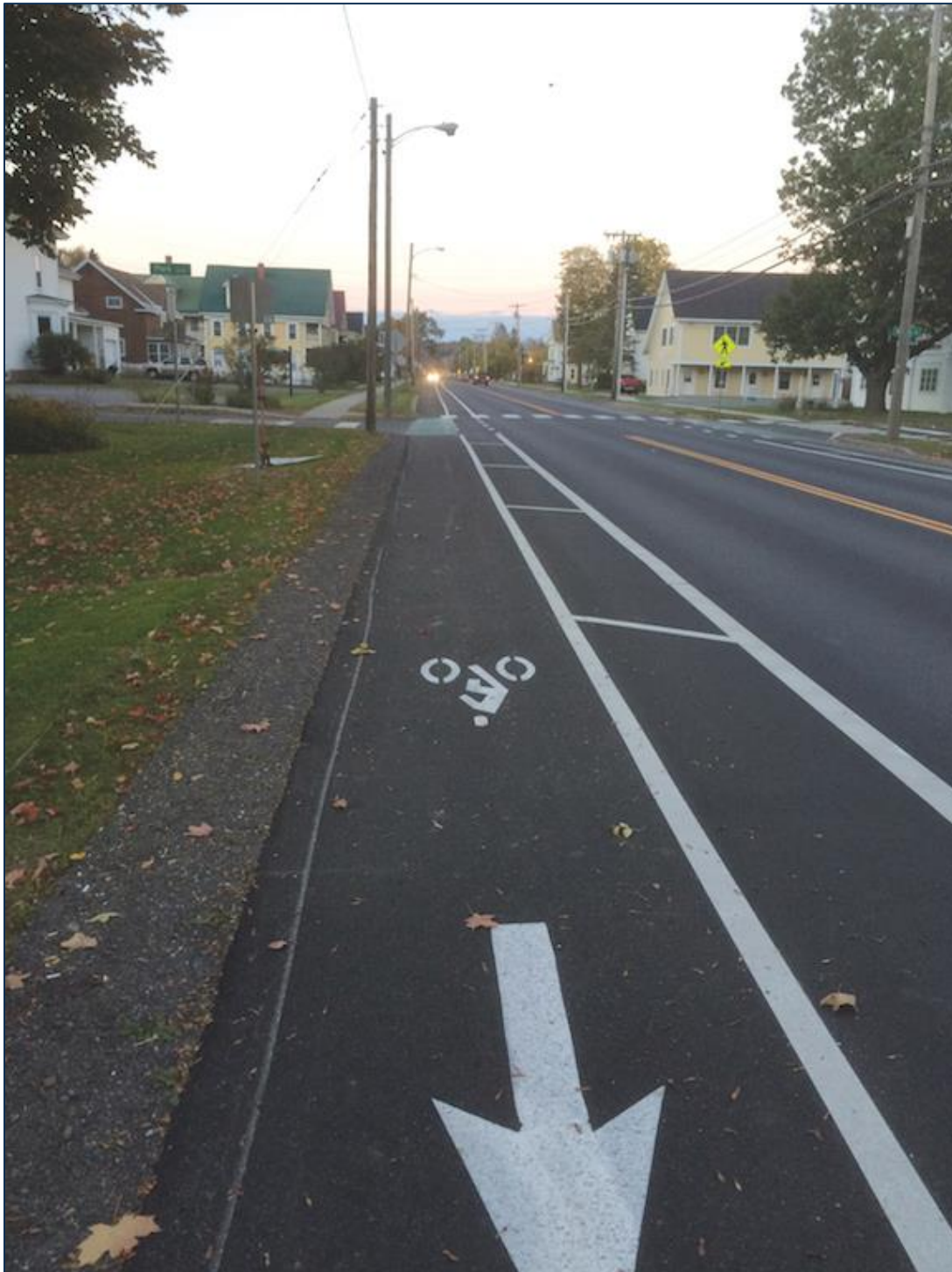
Figure 5.7. City street with visually separated bike lane
