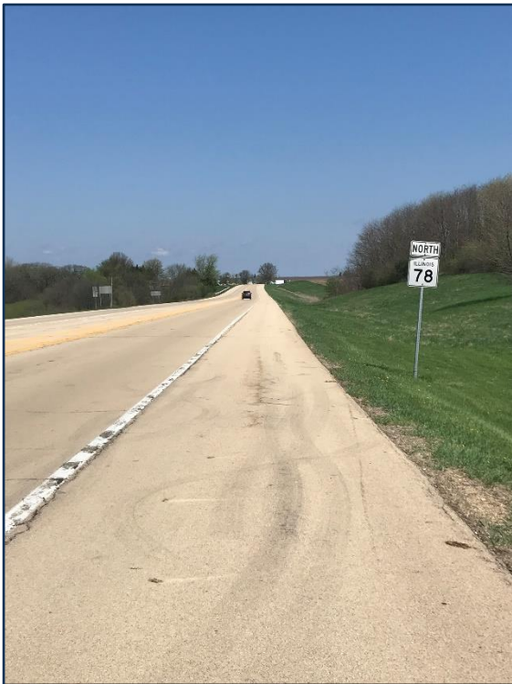
Paved shoulders on Illinois Route 78
