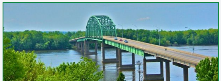
Norbert F. Beckey Bridge
