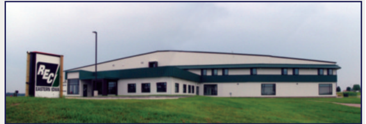
Eastern Iowa Light & Power Cooperative
