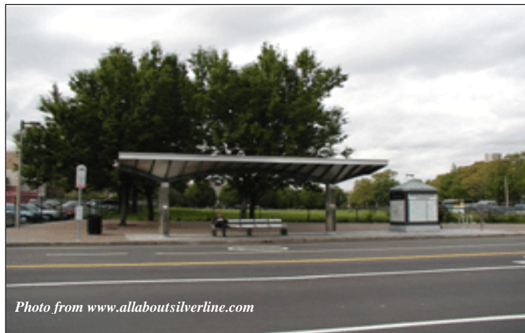
Figure 4 MBTA Silver Line – Melnea Cass Boulevard Station
